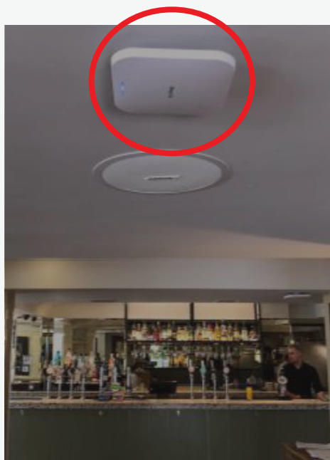
Indoor Access Point
